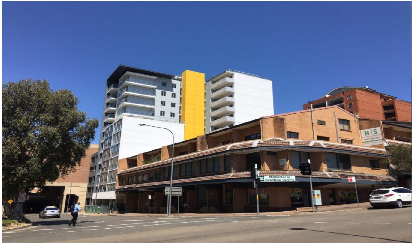
2 VIEW FROM CNR AIRD ST TOWARDS SITE
