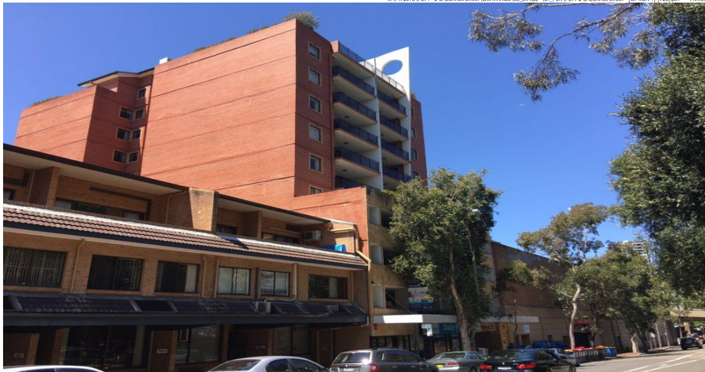
1 VIEW FROM CNR CAMPBELL ST TOWARDS THE SITE
